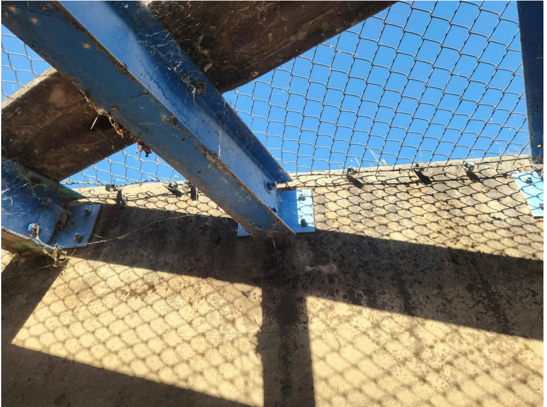
Typical Beam Attachment
