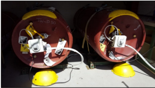
Ton cylinders of chlorine gas
