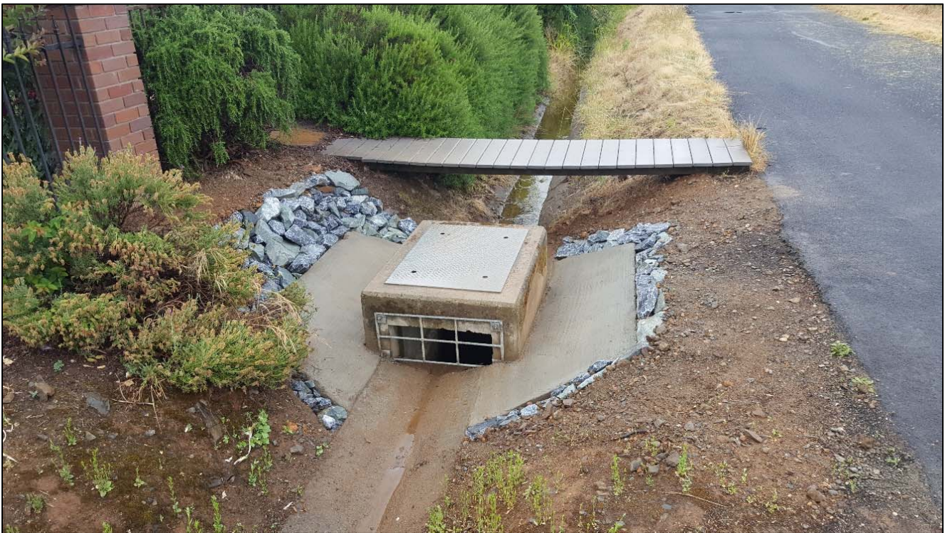
Stormwater inlet repair along the Chesbro protection ditch
