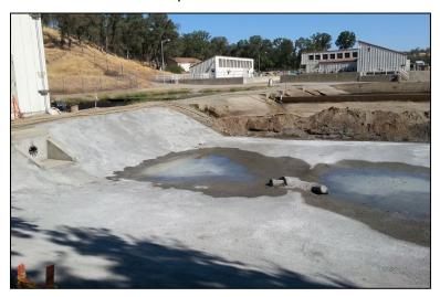
I had staff uncover what is existing to confirm, which is two 4" corrugated landscape drain pipe tied into the "Y" connection that is concreted there. I'm having staff work towards reconstructing it to be as engineered, so it functions correctly.
